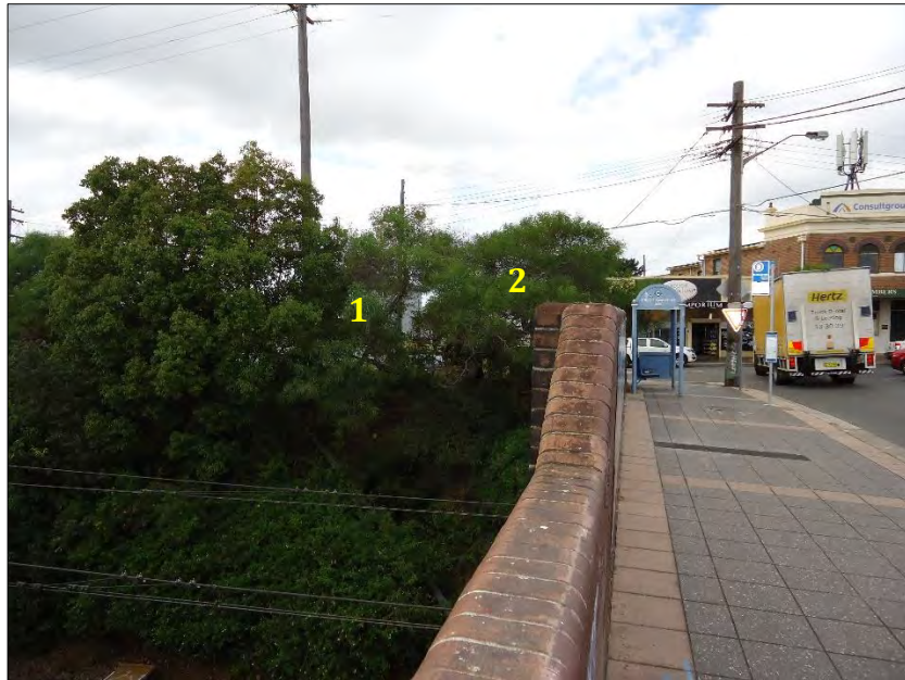
Image 2: Trees 1 and 2, Wattles require removal to accommodate soil pinning works adjacent the bridge.
