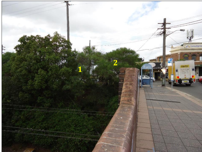
Image 2: Trees 1 and 2, Wattles require removal to accommodate soil pinning works adjacent the bridge.
