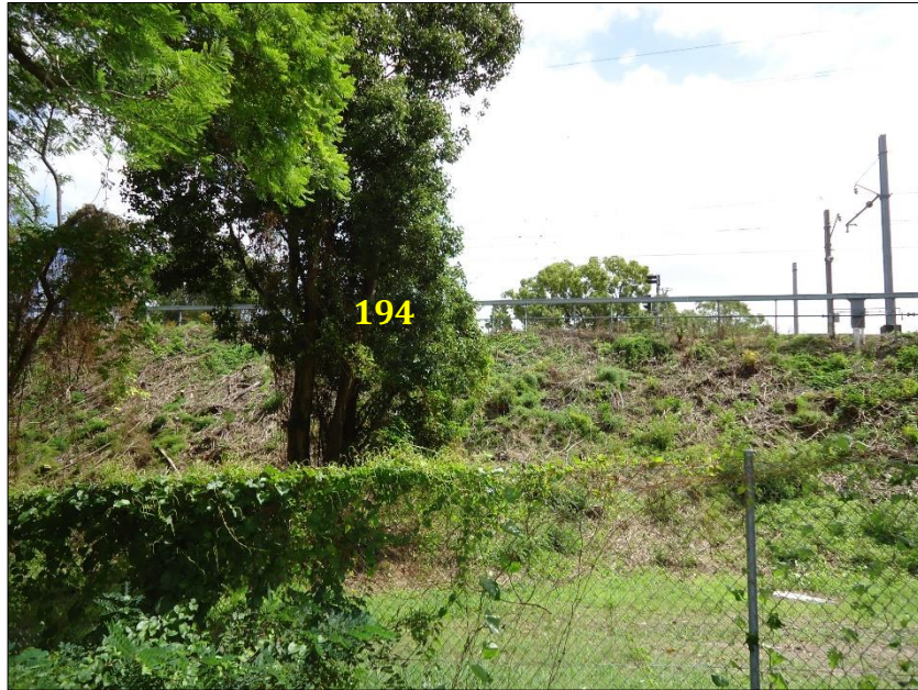
Image 4: Tree 194 as identified within the AIA report shall require removal to accommodate the relocation of the concrete pad. Note the rail embankment to the rear of the tree has been cleared of woody vegetation.
