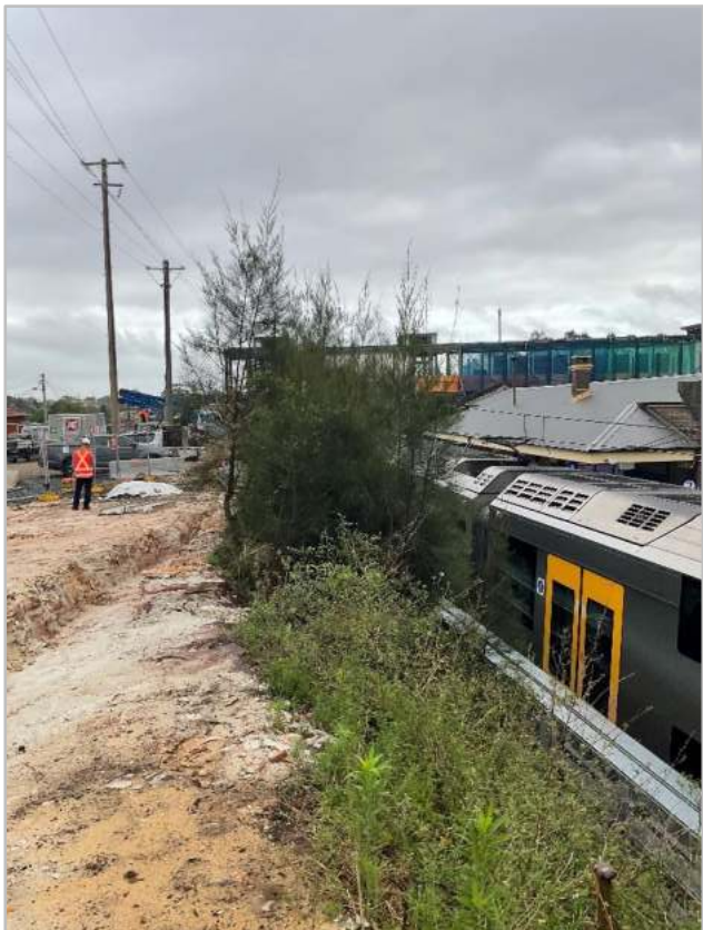
Vegetation within close proximity to infrastructure
