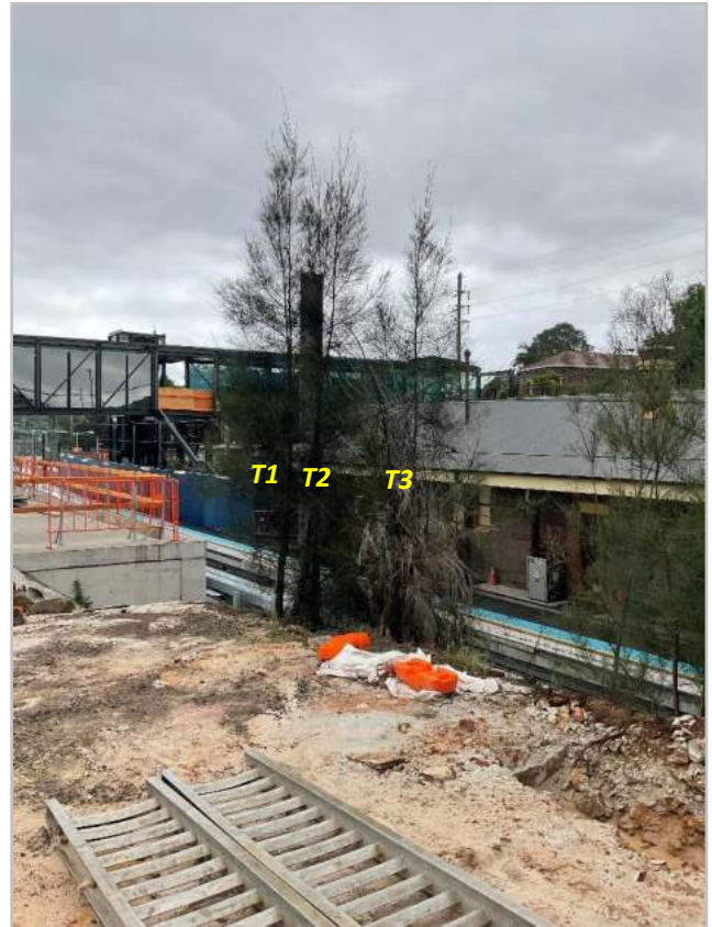
Group of trees needed to clear for trench
