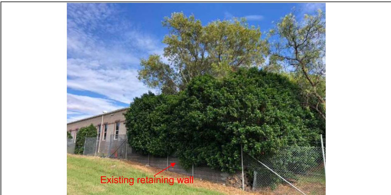
Image 2: Looking towards tree 3316, 3317, 3318, 3319 and 3320, showing the existing boundary retaining wall. The existing boundary retaining wall appears to be restricting root growth into the corridor, therefore, the proposed works within the corridor will not impact the trees. Minor canopy pruning may be required for tree 3316, 3317, 3319 and 3320. The proposed canopy pruning will result in the removal of less than 10% of the live foliage area of the trees and will not significantly impact the trees.
