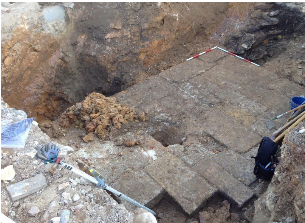
Photo 4 Sandstone pavers uncovered at Balmain East, 2016
