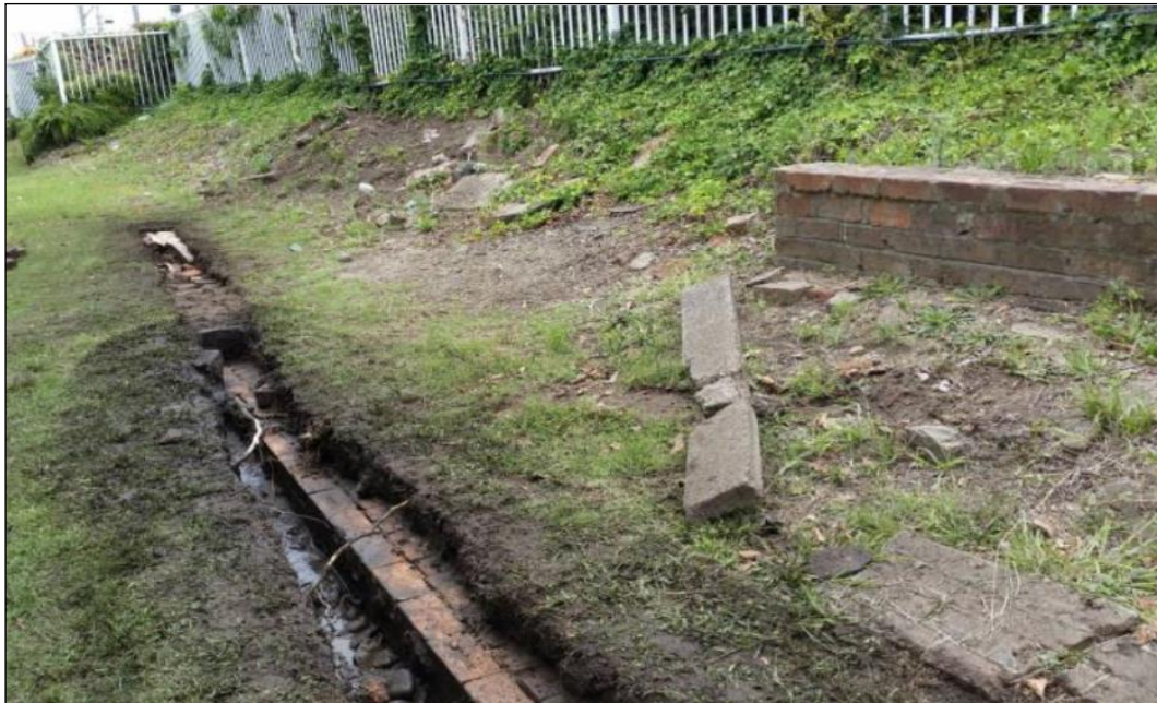
Photo 5 - Platform structure at Hamilton Railway Station classified as a 'work' by the project archaeologist - Wickham Transport Interchange project, 2015
