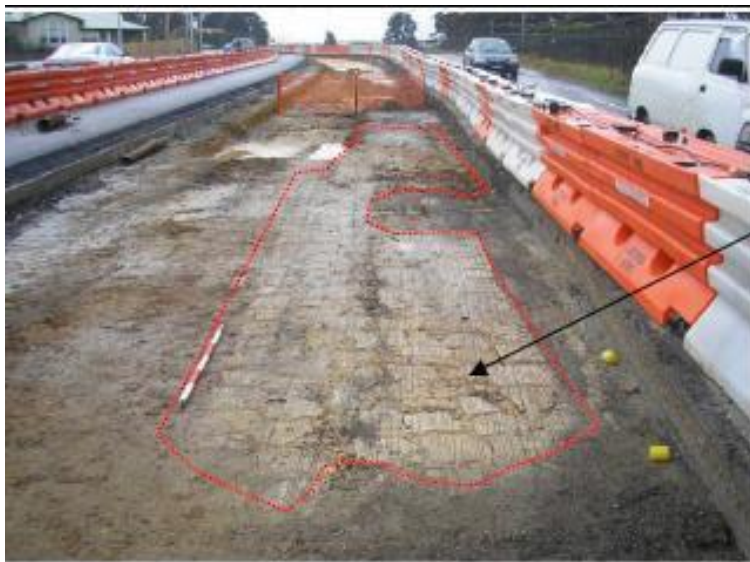
Figure 1: Telford road uncovered on the Great Western Highway (Leura) in 2008 (RMS, 2015).
