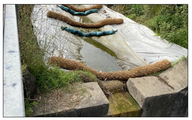
**Photograph 5.** Current condition and sediment / erosion control of the downstream discharge point WP2-DP1 which were located within the rail corridor and immediately upstream / south from WP2 during the monitoring event – 25 August 2022.
