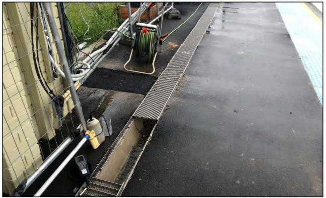
**Photograph 8.** Aco drain check – tap water test. Date: 5 October 2022.
