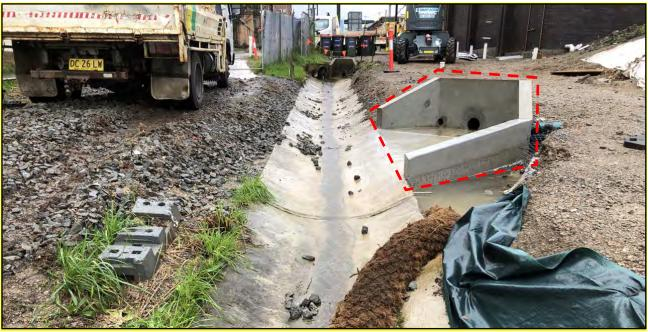
**Photograph 7.** Identified flow contribution to WP2-DP1: platform drainage – stormwater and it was mixed with urban runoff inflow once entering into the concrete lined swale. Date: 21 July 2022.
