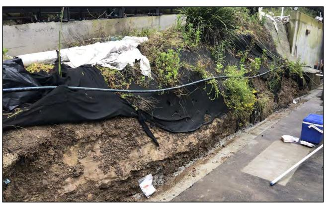
**Photograph 1.** Northern batter – potentially form part of the catchment area to the Platform 1 drainage system. Date: 5 October 2022.
